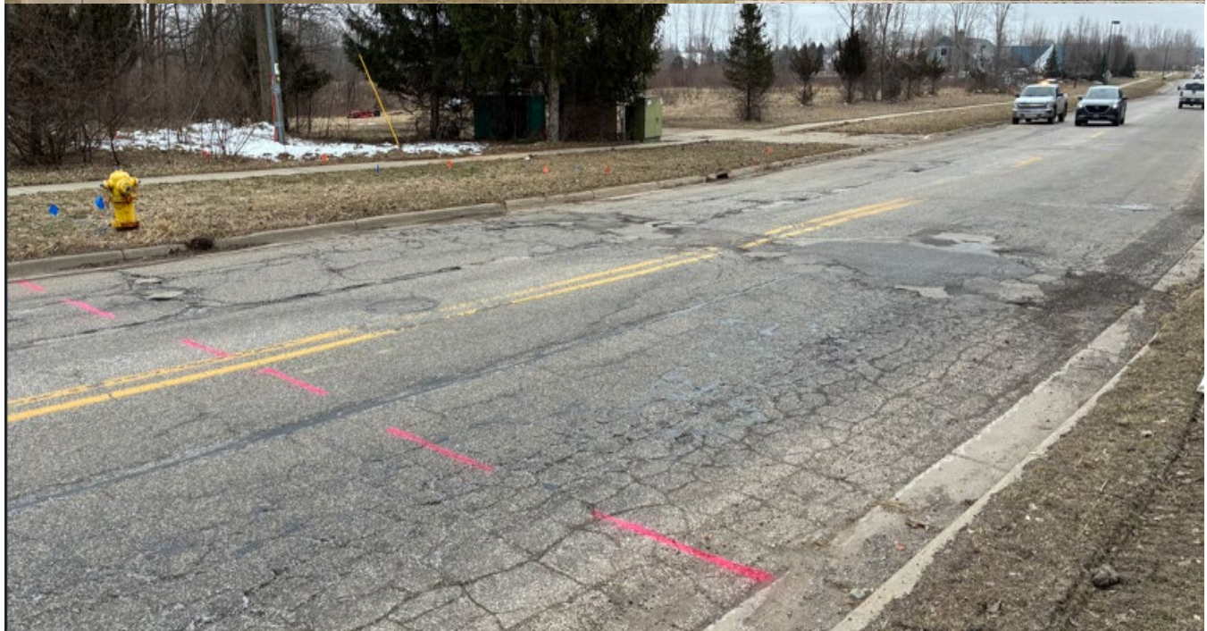
Reno Dr. at curve by LS#7 Both sides of road Approximately 586 square yards
