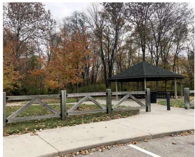
Pavilion at trail entrance.
